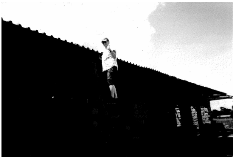
Repairing the school roof in Kenya
